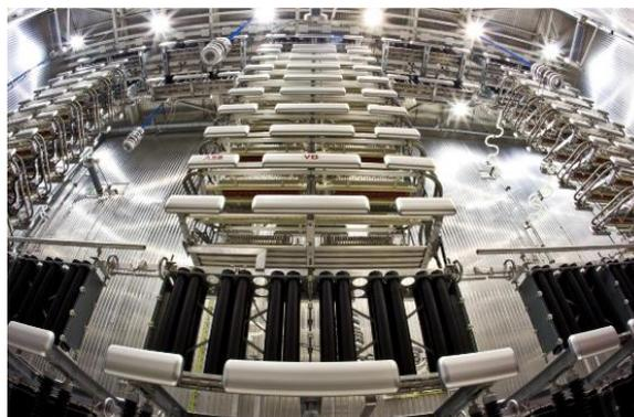
*While converting AC electricity to DC (and vice versa) the valves pictured above switch 1,650 times per second and are controlled via fibre optic cables.*
